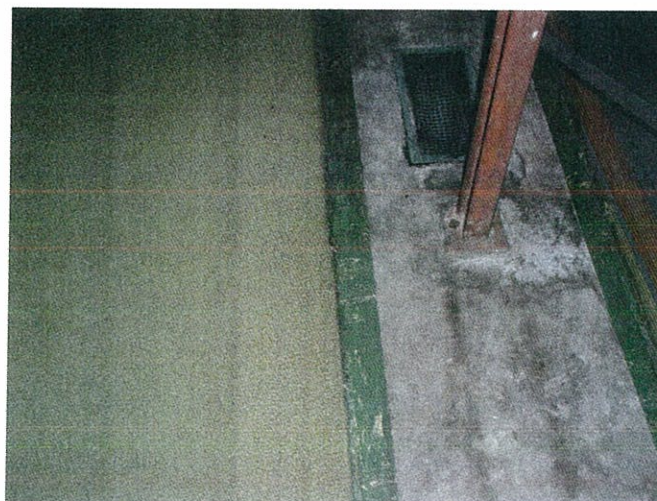
Photo 18: 9-in x 9-in green VFT beneath carpet
