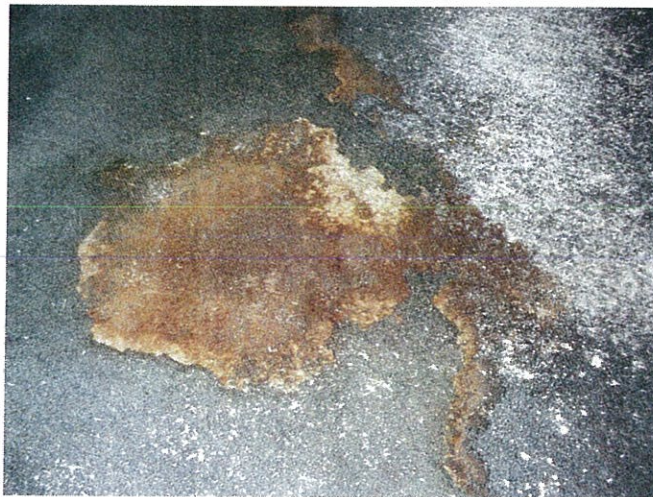
Photo 29: Mold growth on carpeting in Court wing
