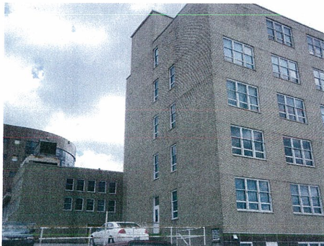
Photo 3: Exterior tower west side
