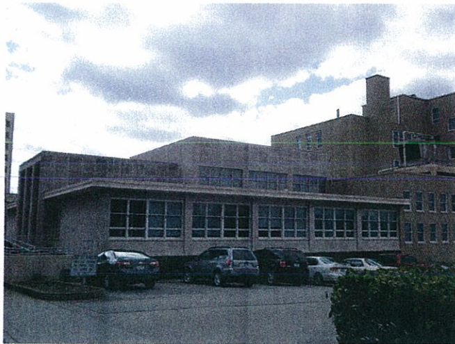
Photo 2: Exterior north side
